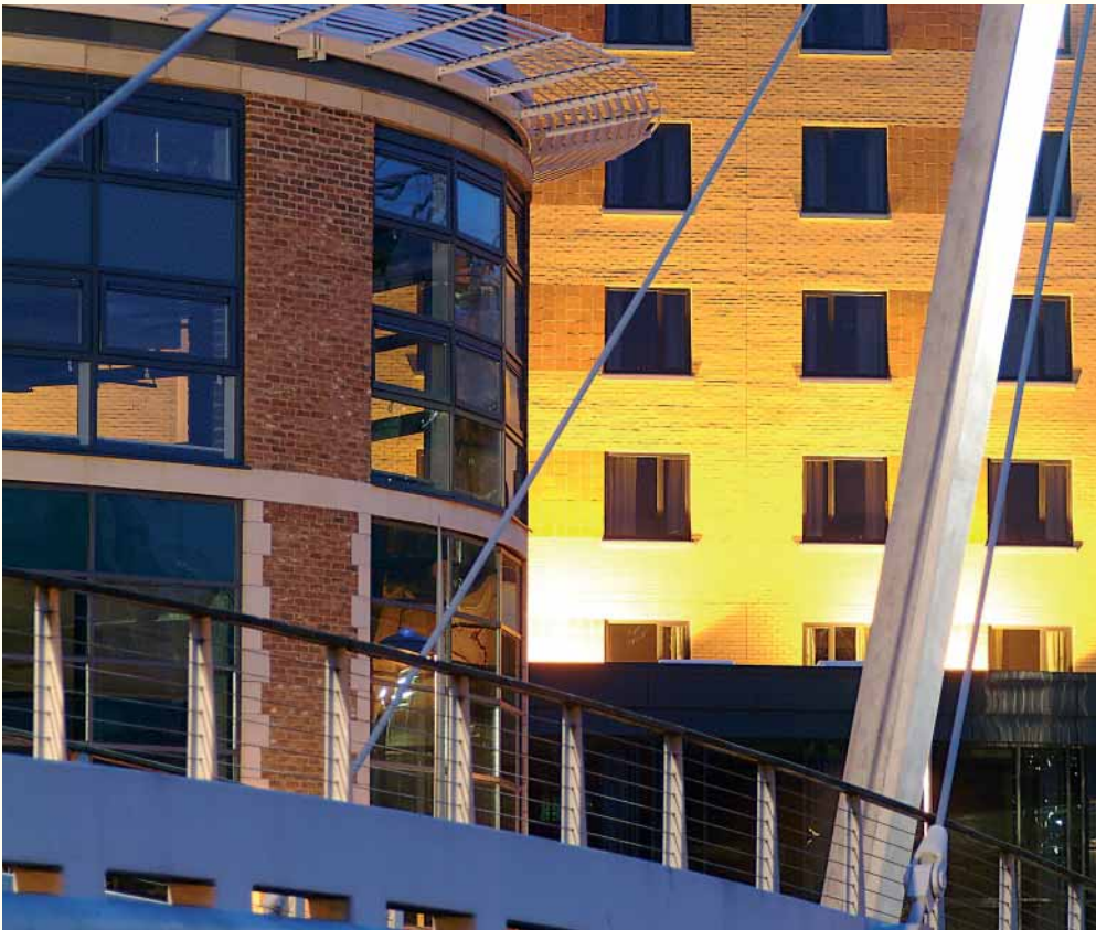
Left Kier Northern undertook the remodelling and fitting out of the Tetley's Brewery Museum at Brewery Wharf, Leeds, to form new offices and retail units.
