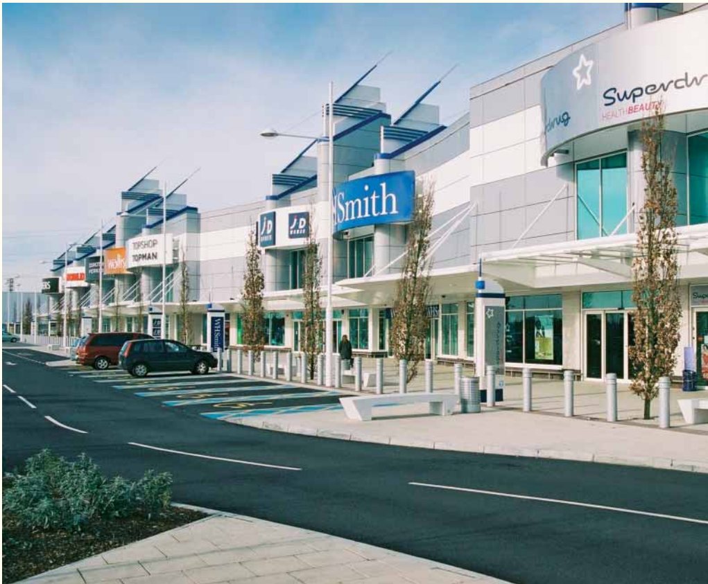
Left A major retail scheme at Beckton by Kier Build, now part of Kier Regional, on land remediated by Kier Construction.
