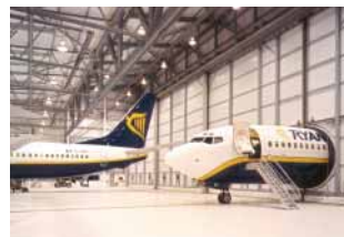
Right A new aircraft hangar facility at Glasgow Prestwick International Airport built by Kier Scotland for Ryanair.
