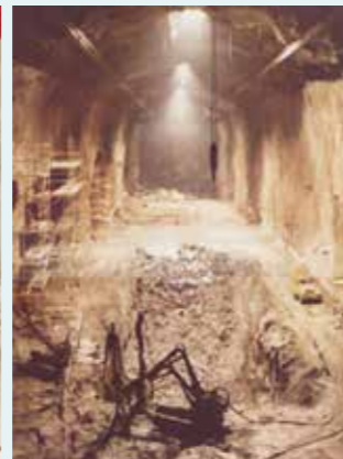
Machine hall incomplete
