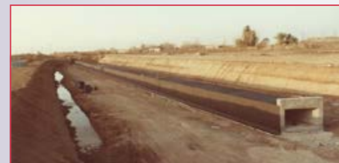
One of the very long drainage culverts under the motorway
