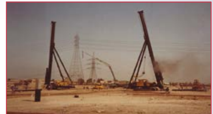
Piling rigs driving pre-cast piles manufactured on site
