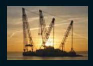
The South Hook project used a 3,300 tonne capacity shearleg crane to remove sections of the old structure.
