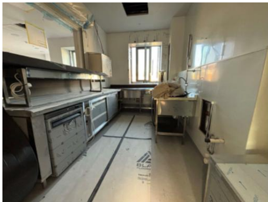
Fresh cook kitchen servery fitting out
