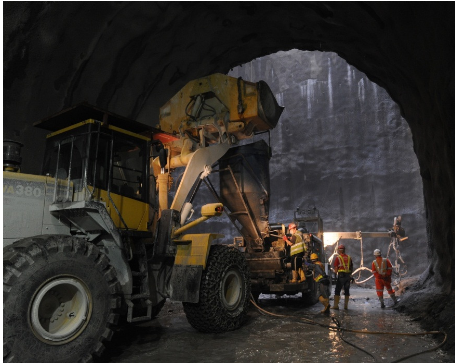
Ngau Tam Mei to Tai Kong Po tunnels, Hong Kong
