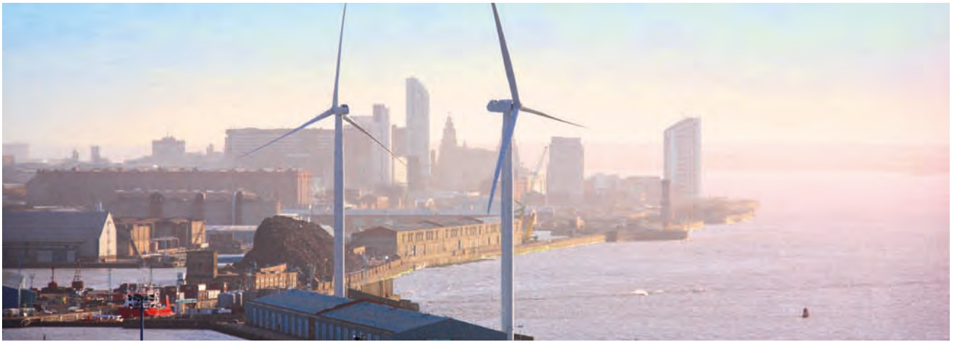
Port of Liverpool Wind Farm, Kier North West
