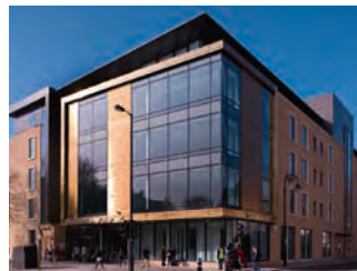
Westminster Kingsway College, Kier London Westminster Kingsway College is a two-stage £35m design & build contract for the provision of a new campus building on one of the current college sites.
