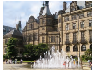
Sheffield Town Hall Kier Asset Partnership Services (KAPS) KAPS achieved its first success in winning a seven-year, £60m contract to manage Sheffield City Council's corporate property portfolio, which started on 1 July 2009.
