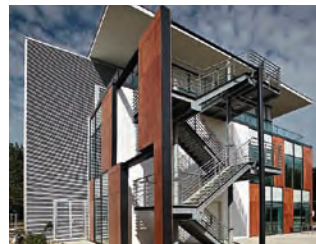
Foundation Park, Kier Moss As part of a £6.5m phased redevelopment, Kier Moss transformed units 7 and 8 of Foundation Park, Maidenhead. The contract included a comprehensive refurbishment and extension to the existing buildings, now occupied by client FREP (Maidenhead) Ltd, and achieved a BREEAM 'Very Good' rating.
