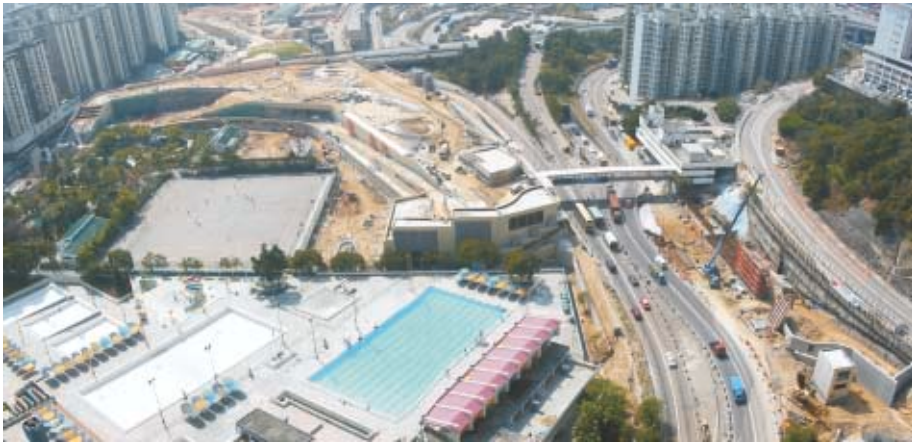
ABOVE Contract 404 Mei Foo Station, a Kier-Zen Pacific joint venture in Hong Kong. Kier Construction.
