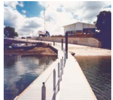
ABOVE New slipway for Ponsharden Marina. Kier Western. 20 21 22 23 24
