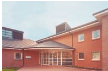
ABOVE Dykebar Hospital for Renfrewshire & Inverclyde Primary Care NHS Trust, Paisley. Kier Scotland. 18
