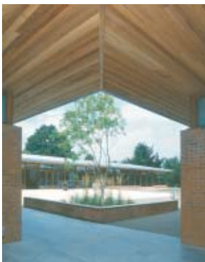
ABOVE Hilliers Arboretum visitor centre, Romsey, for Hampshire County Council. Brazier Construction. 2
