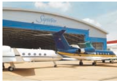
ABOVE New Hangar for Signature Flight Support, London Luton Airport. Marriott Construction. 26 27
