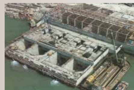
The pumphouse nearing completion
