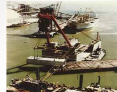
The 'Proteus' heavy lift dry dock barge lowering a single PC Culvert unit onto a barge for transportation to site
