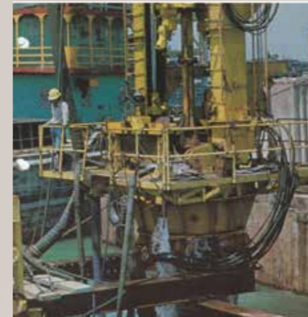
Wirth B6 reverse circulation drilling rig forming piles for pumphouse
