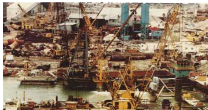
Installation of piling and cofferdam utilising floating plant
