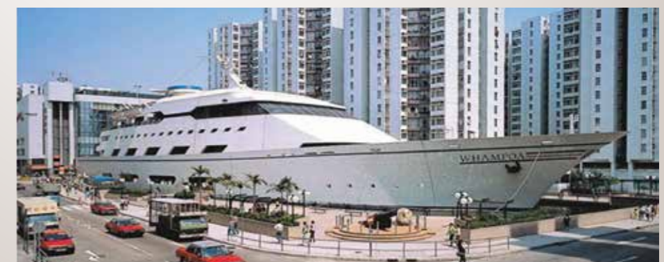
Whampoa shopping centre built in the Hung Hong dry dock, after the KGJV vacated the site
